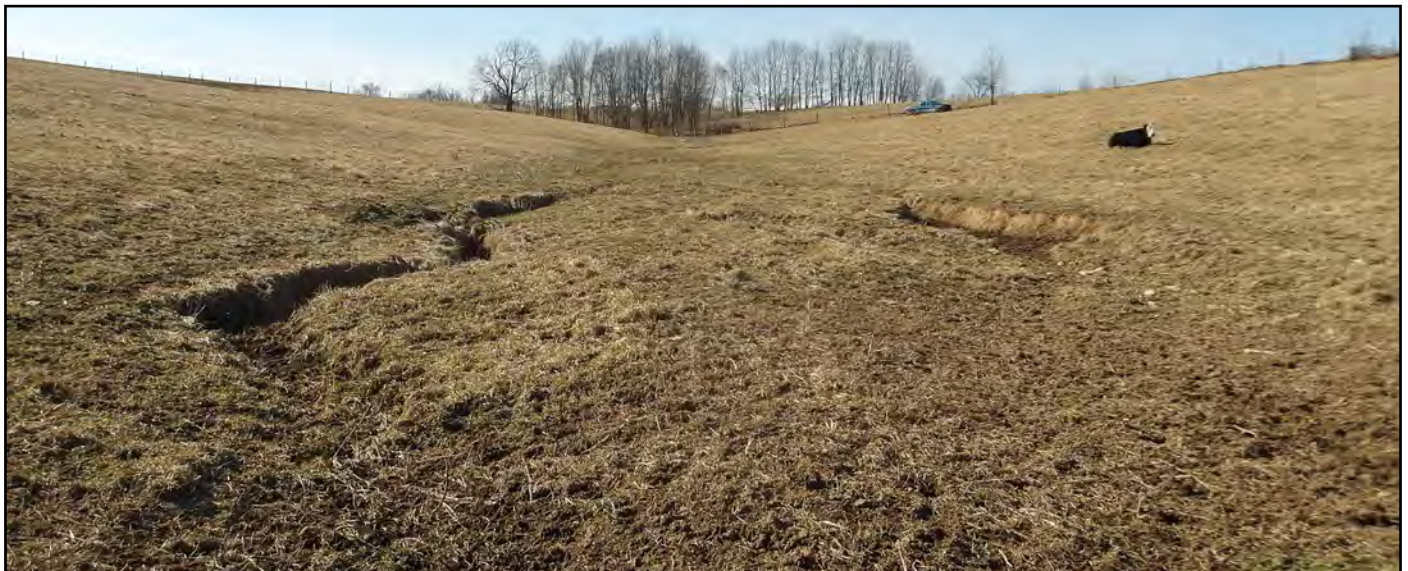
Photo 5: Typical photo of a swale between two hills with eroded stream channels.
