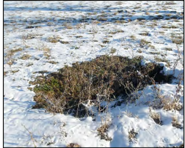
Photo 4: View of a dropout approximately 4 feet wide and 2 feet deep
