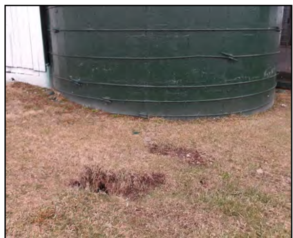
Photo 2: View of a small dropout beside a silo on the south end of the site
